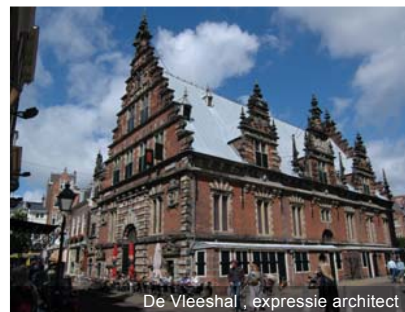
De Vleeshal, expressie architect
